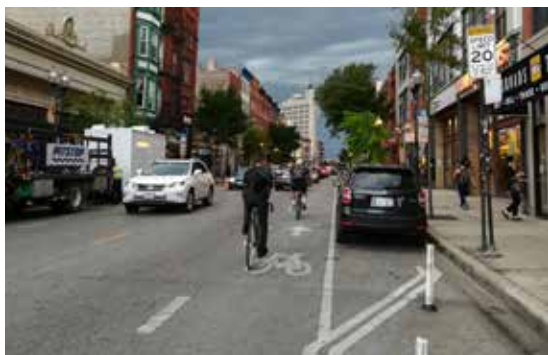
Milwaukee Avenue HCC with a 20 mph speed limit.
