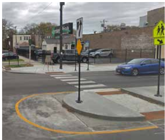
Refuge island and bump-outs installed at Cicero Avenue and Barry Avenue in conjunction with an Arterial Resurfacing project.
